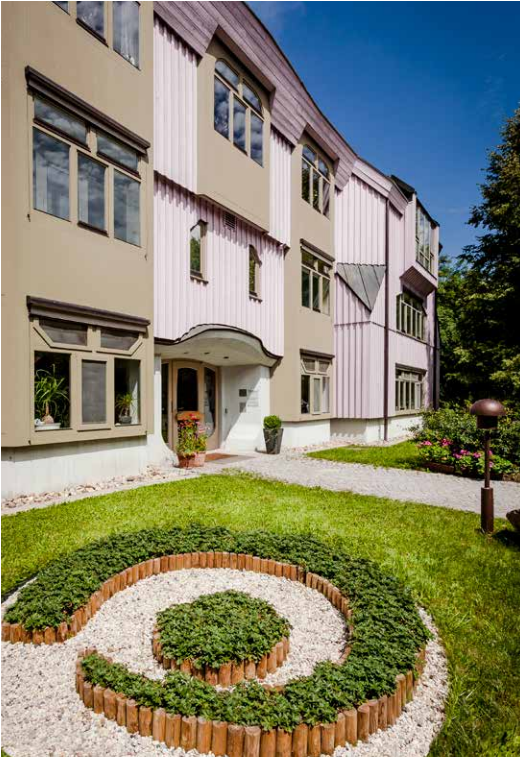
The production building at the Fischermühle in Rosenfeld, Germany
